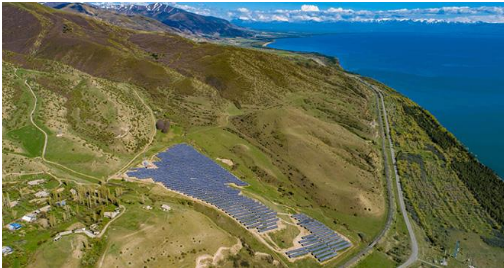
Fig. 4. 5.78 MW solar PV station near v.Tsapatagh, Armenia
